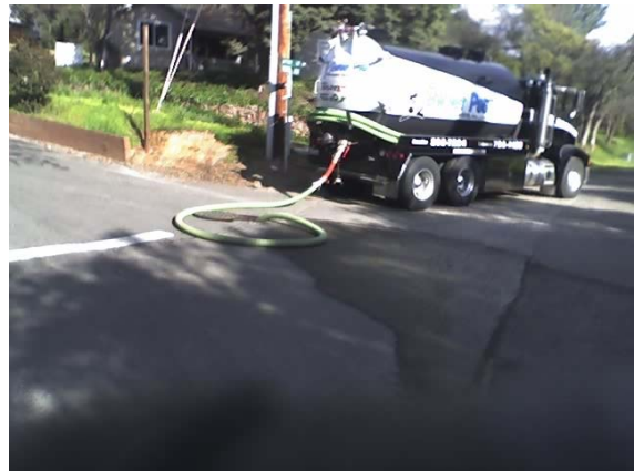
1713 hrs, Manhole # 3744, pumper truck still in position to prevent further overflow.
