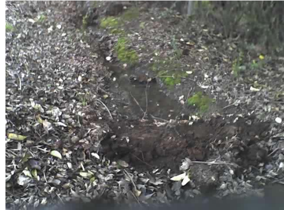
1752 hrs, below culvert outlet S. side of Foothill, with second temporary dam pictured.
