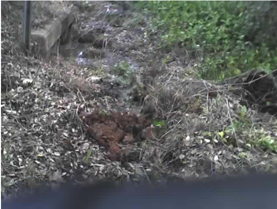
1751 hrs, culvert outlet S. side of Foothill, with temporary dam pictured.
