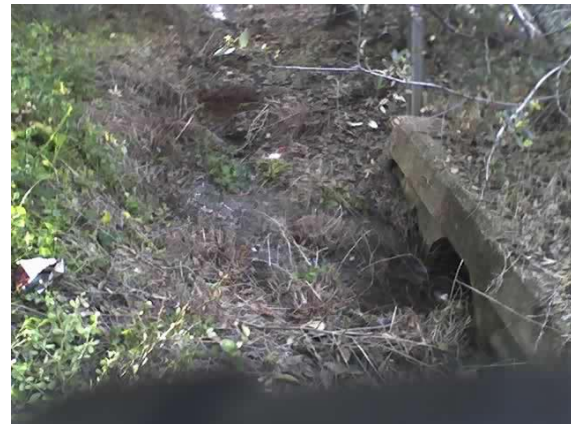
No time noted, culvert outlet S. side of Foothill, post-pumping.
